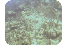
Runway Wall – Poor
